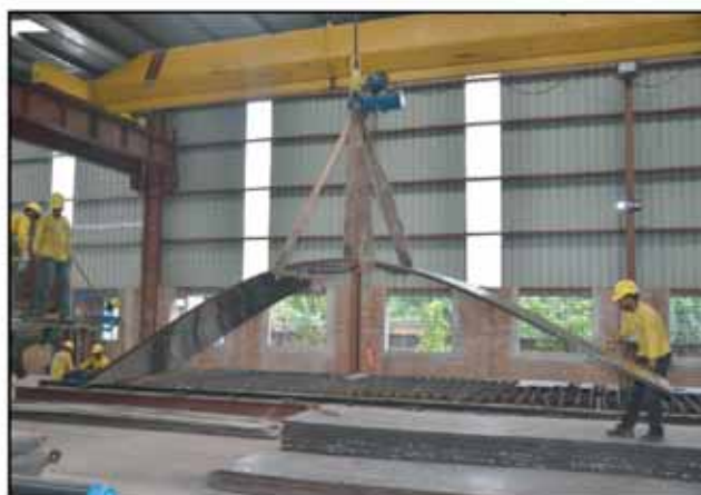
Over Head Crane in Factory
